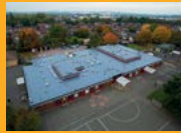
LIQUID APPLIED ROOFING
