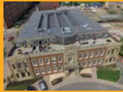
SINGLE PLY ROOFING
