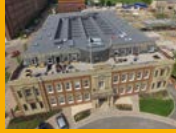
SINGLE PLY ROOFING
