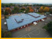
LIQUID APPLIED ROOFING
