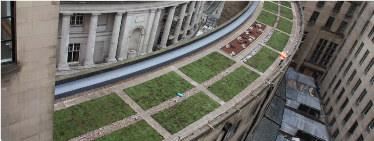
Green roof on Manchester Town Hall, UK.
