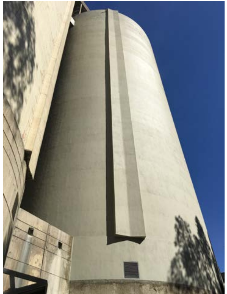
After remedial works.
