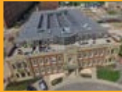
SINGLE PLY ROOFING
