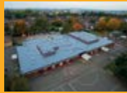
LIQUID APPLIED ROOFING
