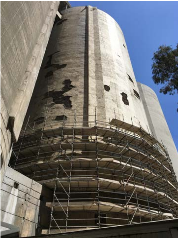
Before remedial works.
